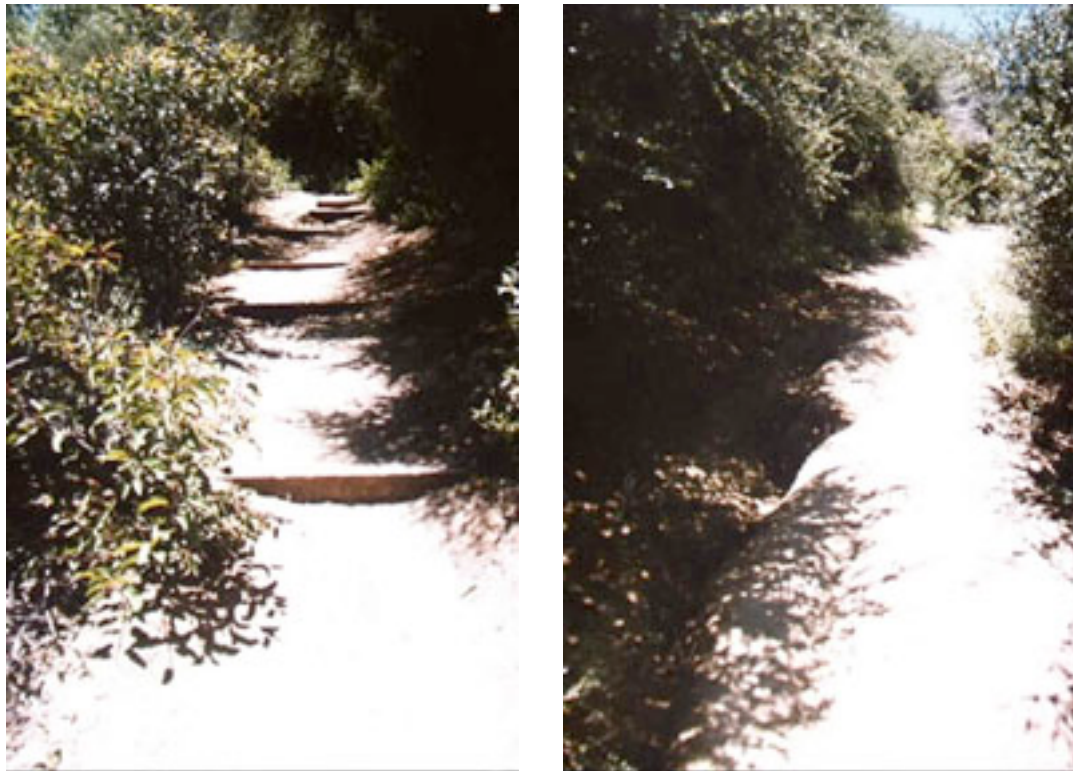
Fig. 7.1 – Set of pictures showing the effect of using water bars on erosion.
